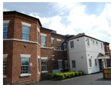
CWP Trust Headquarters at Redesmere
